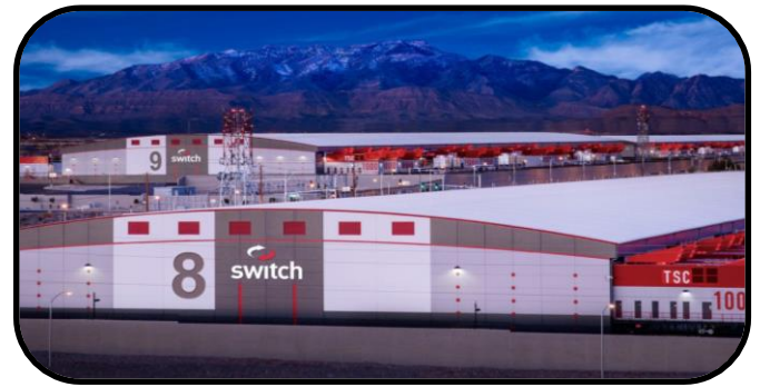
Photo via: Switch, https://www.switch.com/photos/
