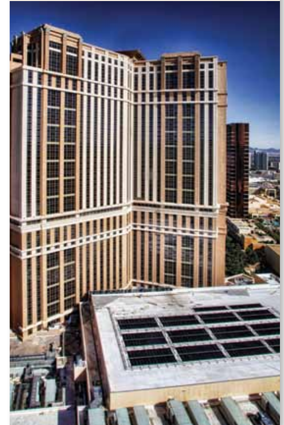
Rooftop solar-thermal system in Las Vegas
