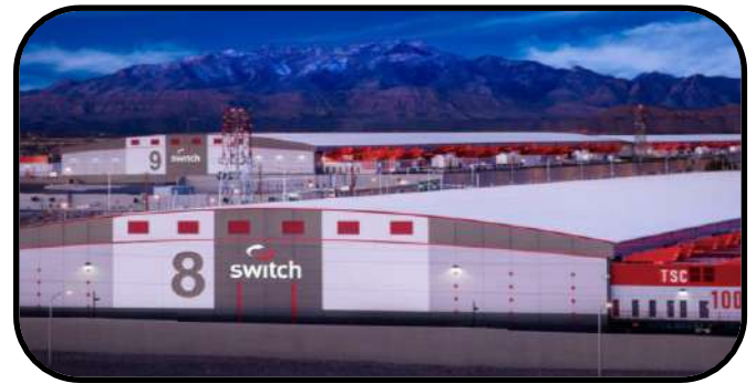
Photo via: Switch, https://www.switch.com/photos/
